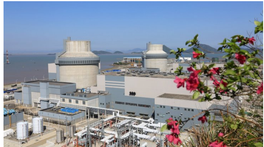
Westinghouse-designed AP1000s at Sanmen, China (Image: Westinghouse)
